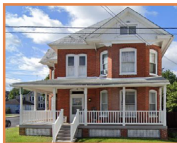
102 N Queen St - Littlestown
